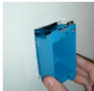
Various interconnect methods can be used. The conduit may be rigid or flexible metallic or non-metallic type. Some clients choose to install without conduit by using the low voltage in-wall wiring solutions. The mounting boxes may be regular in-wall, low voltage drop-in boxes, or surface mounted boxes.
